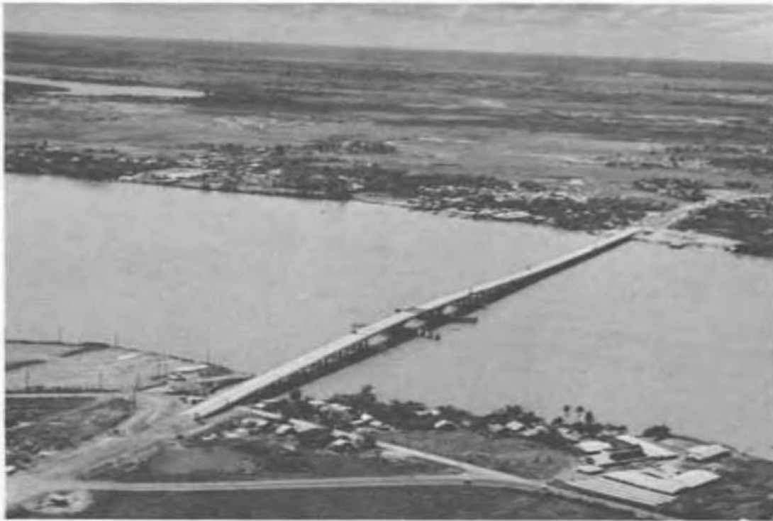
53. Bien Hoa Bridge. This is the largest of the 6 bridges which comprised a major bridge building program ($20 million) in the Saigon area. The Bien Hoa span is 2,631 feet long; it crosses the Dong Nai River on QL 1, 17 miles northeast of Saigon. It was started on 15 May 1971 and was completed on 1 May 1972, at a cost of $4.5 million.
